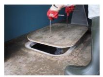
Check the compost pile for "peaking" and if required use the rake stored in this vault to bring the pile towards the front (door) end of the vault. This prevents excessive build up of compost directly below the toilet which could ultimately impede the function of the urine gutter. At no time should the compost be closer to the urine gutter than about 100mm. This operation also helps to bring the pile into the final position for emptying after the vault resting period.
