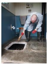
Raking the compost towards the door end and sweeping the flange before refitting the hatch.
